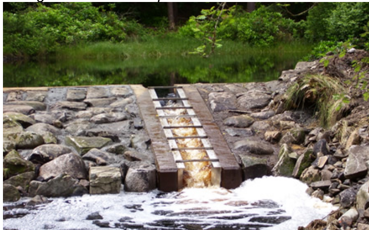
Figure 12: Denil fish pass fitted on the Polbae Dam
